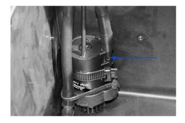
Finished product should look similar to this. Once the pump is turned on, water will spew out of hole, allowing any airlock to be purged from the system as well. Reverse steps to reinstall the pump shroud\*
