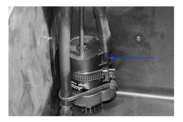
Drill a small pilot hole (1/16th) in the location indicated by the arrow. Next, drill 1/8th" hole in pilot hole location. Be sure NOT to drill through both sides of tube, hole only needs to be in the outer side of the tube
